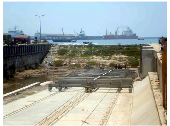
Slipway upper/lower cradle combined going down
