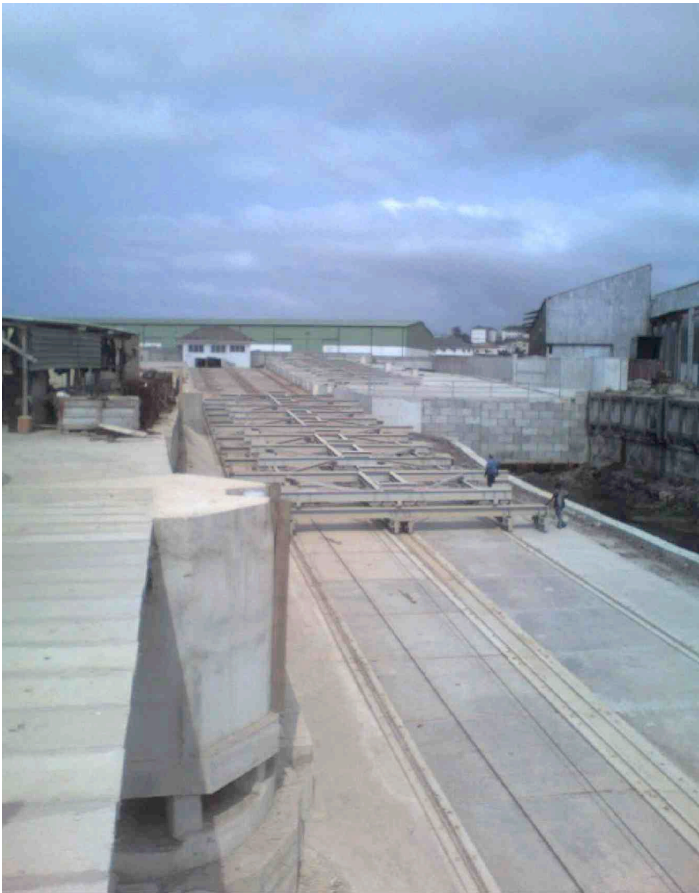
Slipway lower cradle going down
