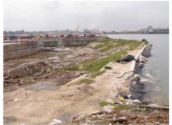
Temporary cofferdam with sand bags
